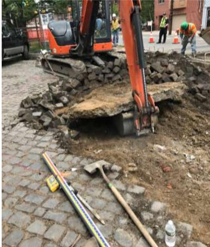
Photograph 7 – View of excavator lifting 6-inch concrete level underlying Belgian Block cobbles, taken facing northwest.
