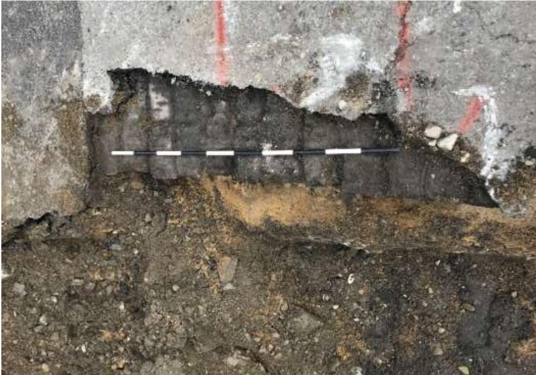
Photograph 5 – Overhead, or plan, view of the eastern edge of the trench showing the Belgian Block cobbles continuing under the asphalt pavement surfacing Paterson Avenue.
