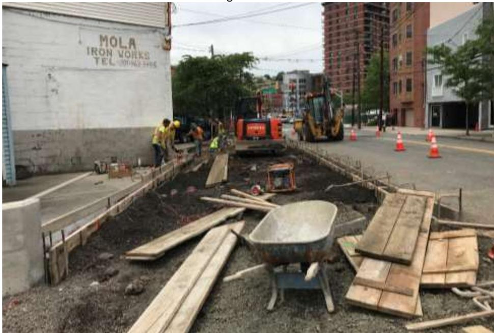
Photograph 8 – View of the completed excavation for the 15-foot wide sidewalk with two curbs paralleling Paterson Avenue, facing northwest.
