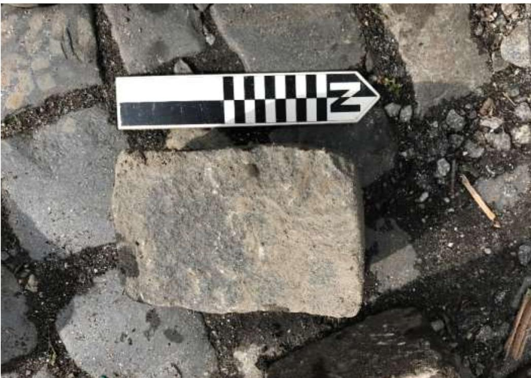
Photograph 6 – Overhead view of a single Belgian Block used for the cobbled surface.
