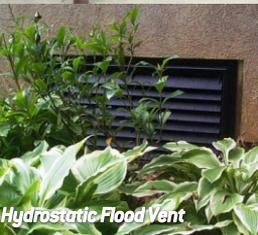
Hydrostatic Flood Vent
